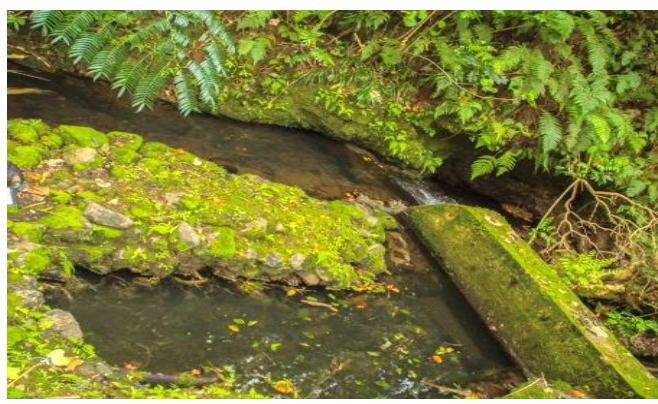
One of three open intakes , the Totokoitu intake, and water is collected directly from a side basin created beside the stream. Other intakes with the same filtration system are Papua and Muriavai – Photo by Jahz Photography
