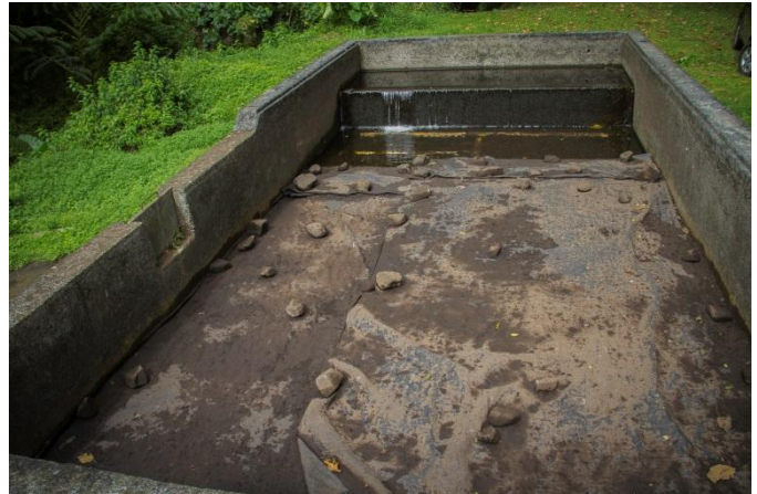
Figure 12 - Two filtering systems used at the intakes (Left: Tupapa (for the fine objects) and tot he Right is at Ngatoe (for large objects))
