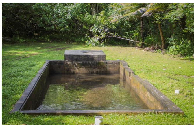
An example of an Off-stream Rapid filtration and this one is at Ngātoe intake. It removes most solids and some organic matter. Other intakes with the same filtration system are Tupapa, Matavera and Rutaki – Photo by Jahz Photography
