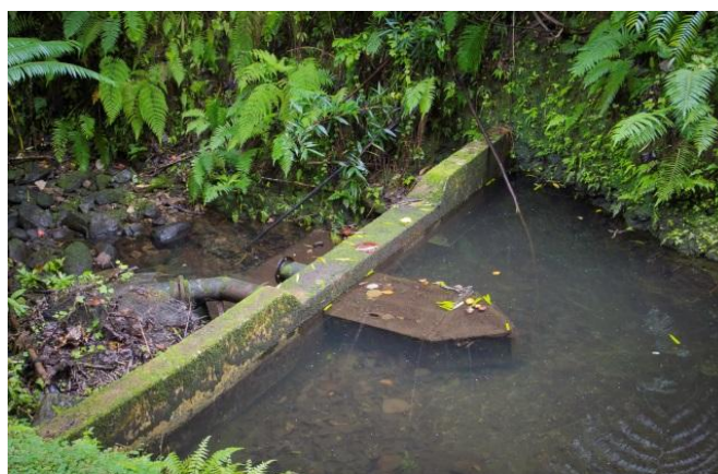
An example of a Filter at Ngātoe Stream to remove gravel, sticks and large objects before water enters the Off-stream filtration – Photo by Jahz Photography
