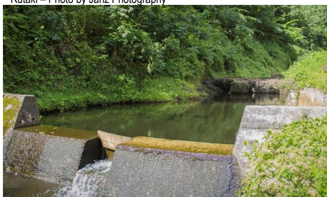
In-stream Rapid Filtration at Avatiu Intake, Turangi Intake, Takuvaine Intake, Avana Intake and Taipara Intake, with a wall of basket of rocks upstream to reduce larger objects from entering the filtration area – Photo by Jahz Photography
