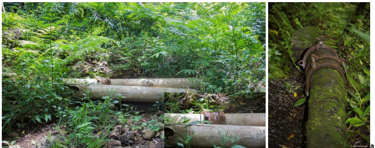
Figure 15 - Right- Pieces of inert asbestos pipes found along the Turangi intake roadside (September, 2014) 2014, Left – A section of asbestos pipe line currently in use, Totokoitu trunk main (September, 2014) -Photos by Jahz Photography
